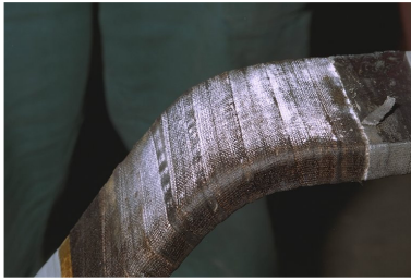
Fig.14: White traces at endwinding due to corona degradation
