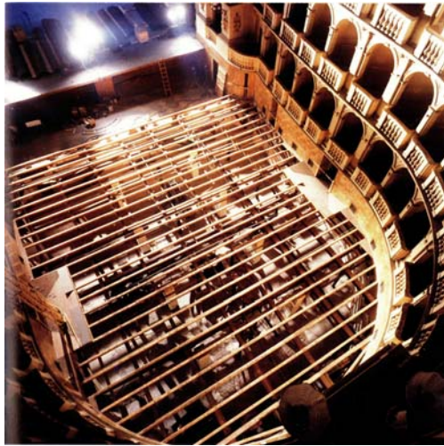
Fig. 1 The cavity below the stalls
