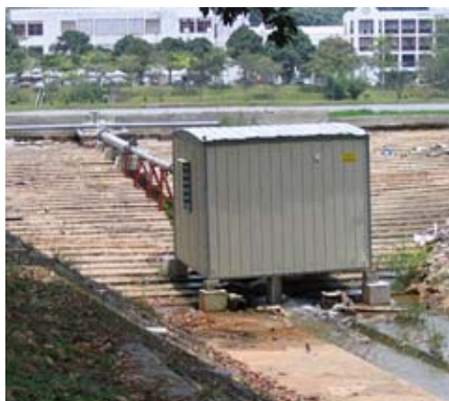
Fig. 3 Pico hydro system in the university lake
