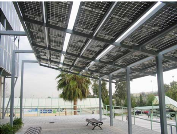
Fig. 6. Photography of ‘Pergola’ system
