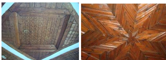
Picture 7. Room Ceiling [16]
