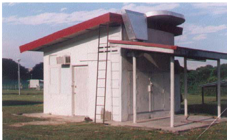
Fig. 2. The photograph of forced convection solar dryer with V-groove collector
