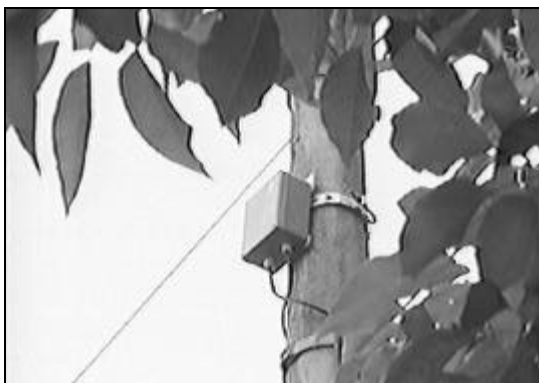
Fig. 4 - Outdoor three-phase unit (for pole installation).
