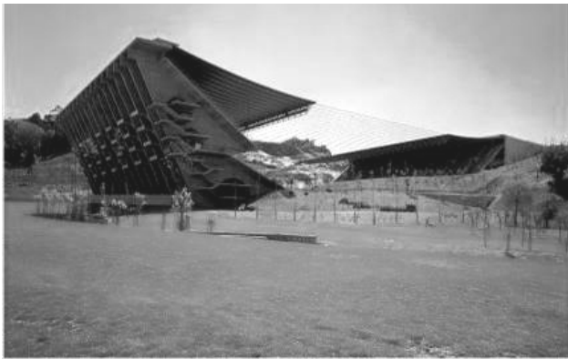
Figure 4- View of the Braga Municipal Stadium and surrounding landscape.
