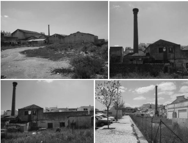
Figure 6- Derelict buildings of the Arade valley old industrial landscape.
