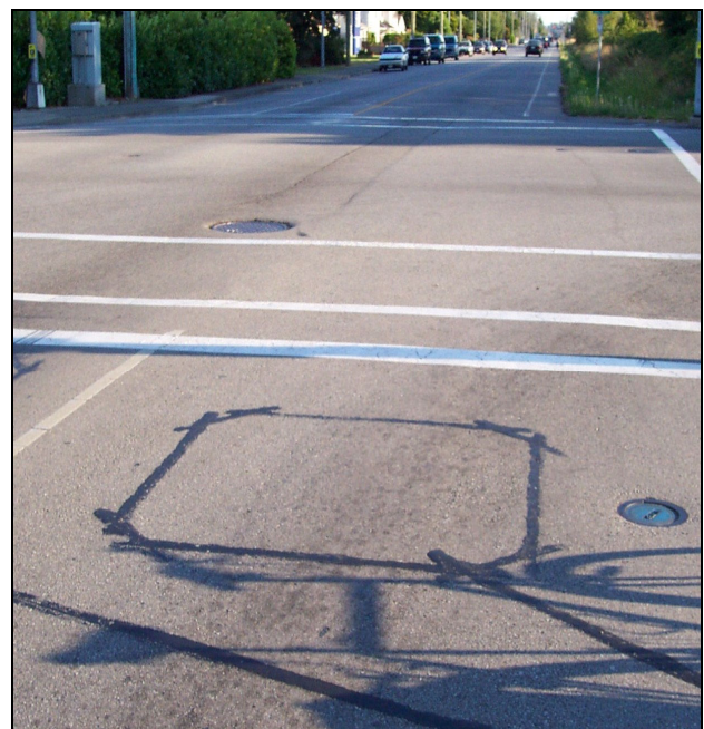
Fig. 3: The magnetic loop sensor placed at the road end before the junction.
