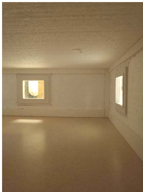
Figure 9: Polystyrene wall and ceiling viewed from inside.
