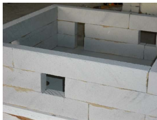
Figure 2: AAC external walls building
