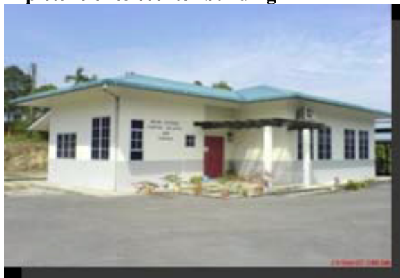
A picture of telecenter building
